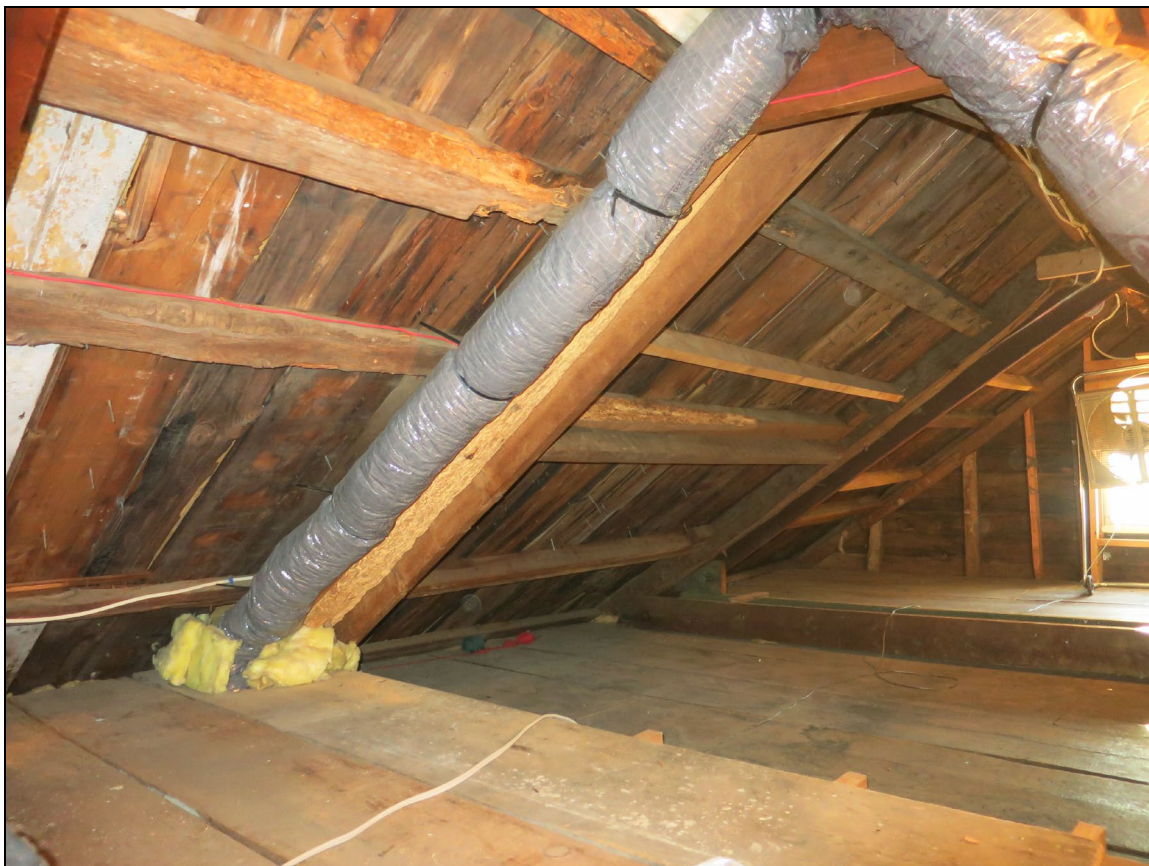
Attic, roof framing.
