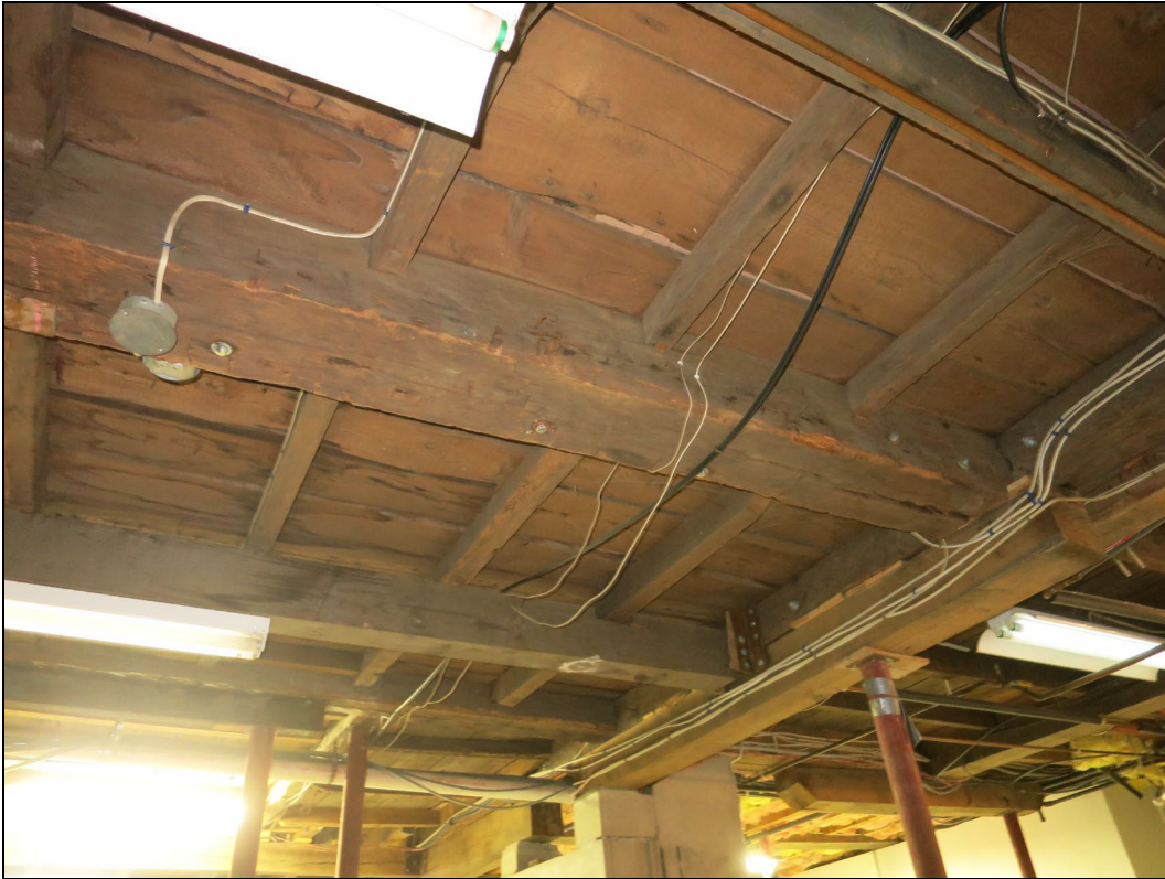
Basement, first floor framing.
