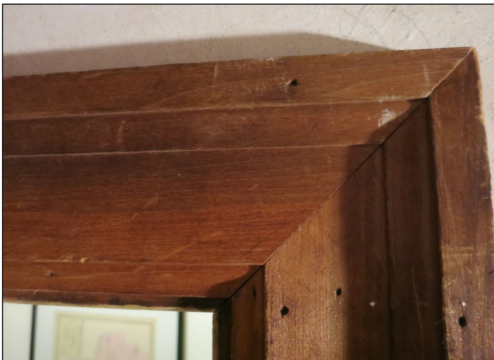
18 th -century trim on inside of door to attic stairs.
