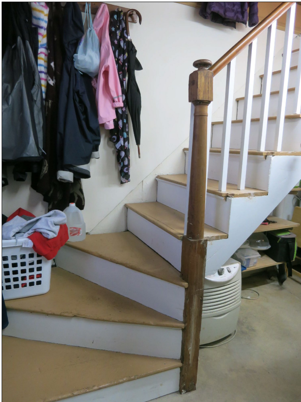
Basement, relocated 18 th -century stair post.
