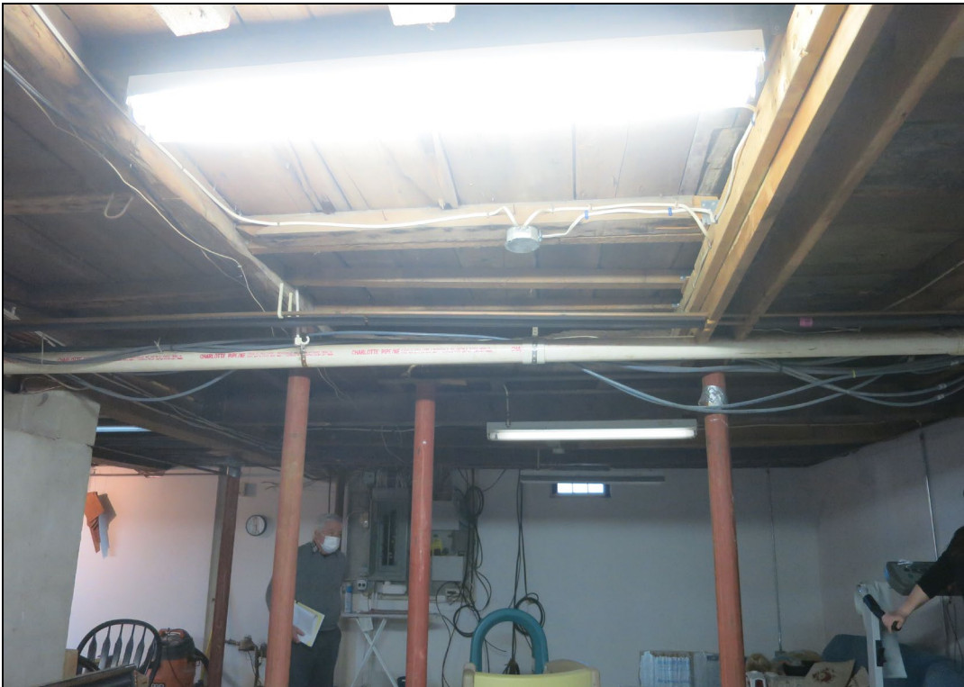
Basement, patched flooring where chimney was removed.
